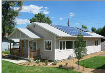
The NREL/Habitat for Humanity Net-Zero Energy Demonstration Home in Wheat Ridge, CO, has exceeded performance expectations, generating a surplus of power in its first two full years of occupation.
