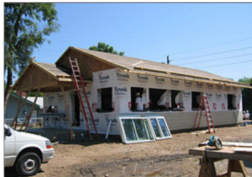
The NREL/Habitat for Humanity Net-Zero Energy Demonstration Home in Wheat Ridge, CO, was built in 2005 with several energy efficiency elements, including three-foot roof eaves, solar-tempering windows, moisture barriers, and extra insulation.
